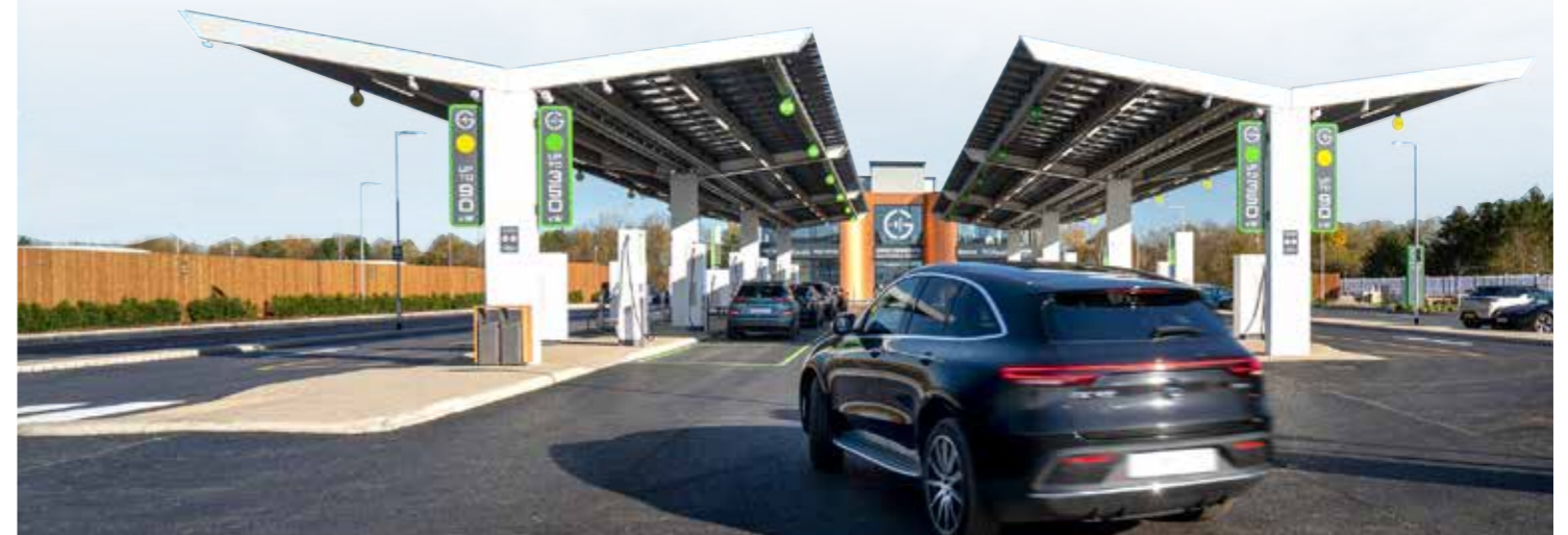
The forecourt deploys ‘sun-to-wheel’ infrastructure with electricity generated from solar power canopies as well as off-site solar farms
