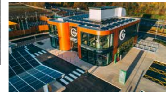
The forecourt deploys ‘sun-to-wheel’ infrastructure with electricity generated from solar power canopies as well as off-site solar farms
